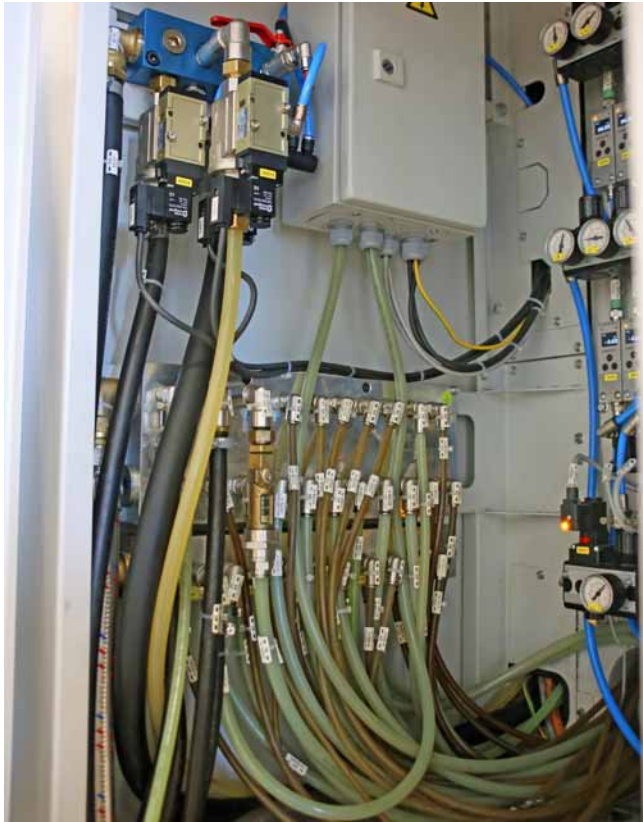
Temperature-conditioning of all key components for the Röders machining centres is a prerequisite for high-precision milling (Photo: Klaus Vollrath)
